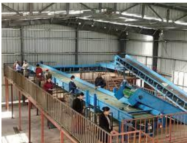
Figure 6: Material Recovery Facilities
