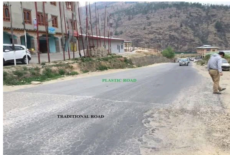
Figure 14: Bhutan's first plastic road, built by Green Road in 2015, is a 150-meter stretch using 555 kg of waste plastics. Completed on October 5th, this durable road has required no repairs, showcasing a sustainable solution to plastic waste and innovative construction.
