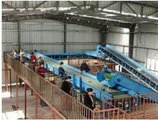
Figure 6: Material Recovery Facilities
