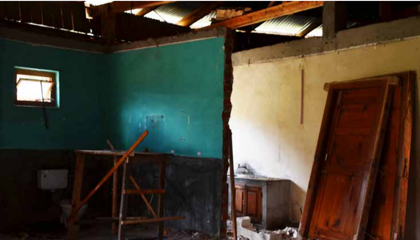
The renovation work under progress
