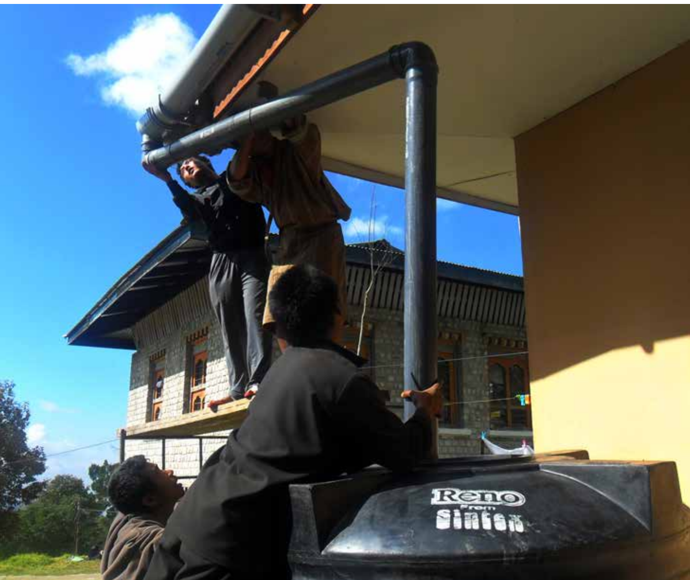
Installation of rain-water harvesting facilities.
