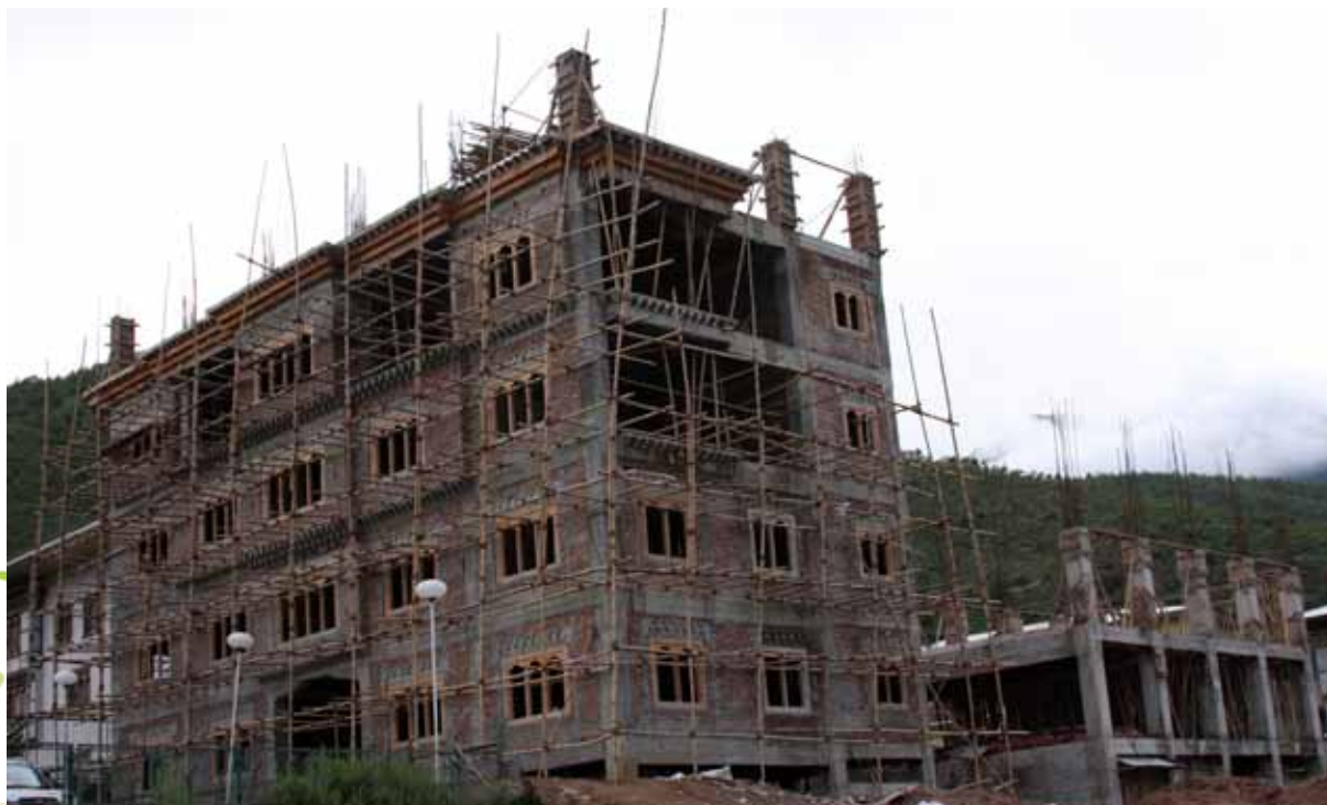
RSPN's headquarter and environmental resource centre under progress
