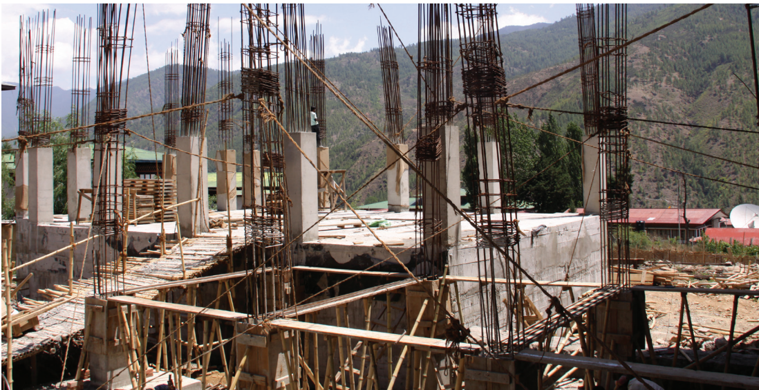
Air and water pollution from unregulated construction increases every year.
