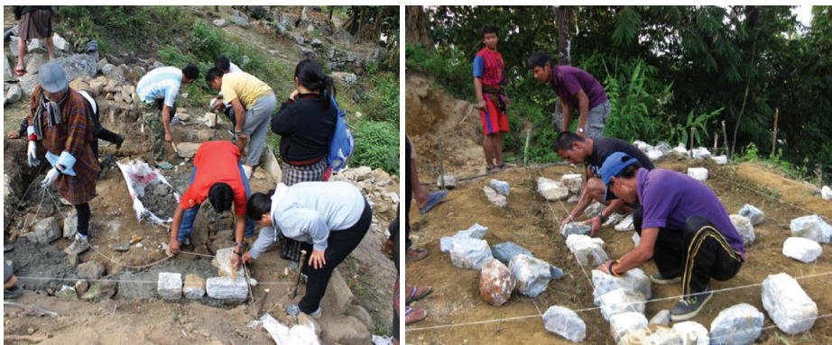
Local community members being trained on basic masonry skills
