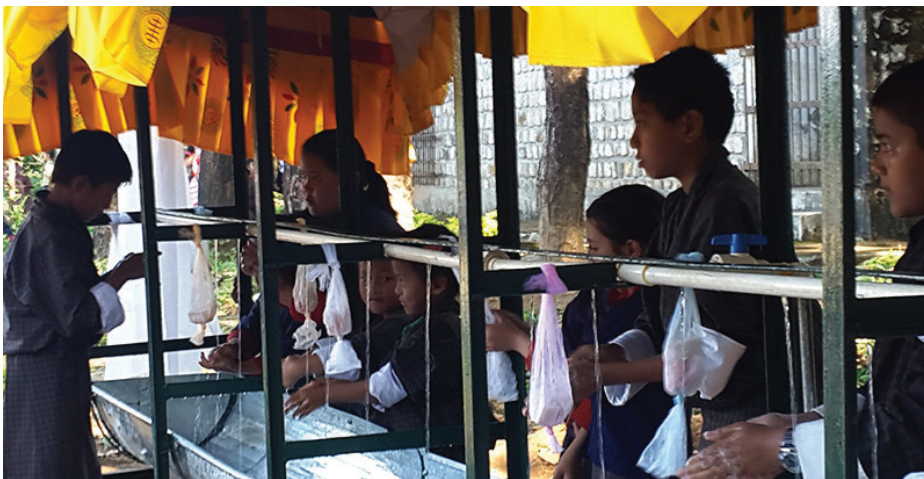
Students wash hands at newly installed facility.
