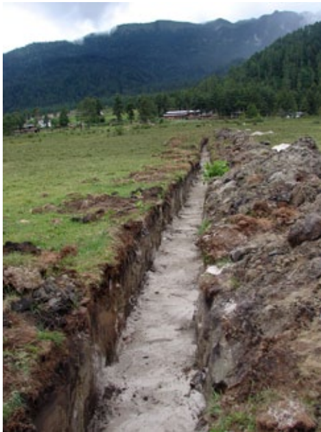
>> Underground cable tunnel under progress
